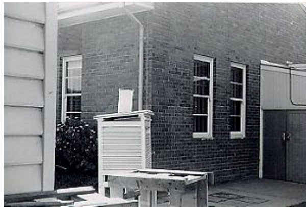
This photo shows the position of the Stevenson screen at the back of the Post Office in Deniliquin. The temperature was sampled at this site from 1873-1971. Note the close proximity of buildings and paved areas.
